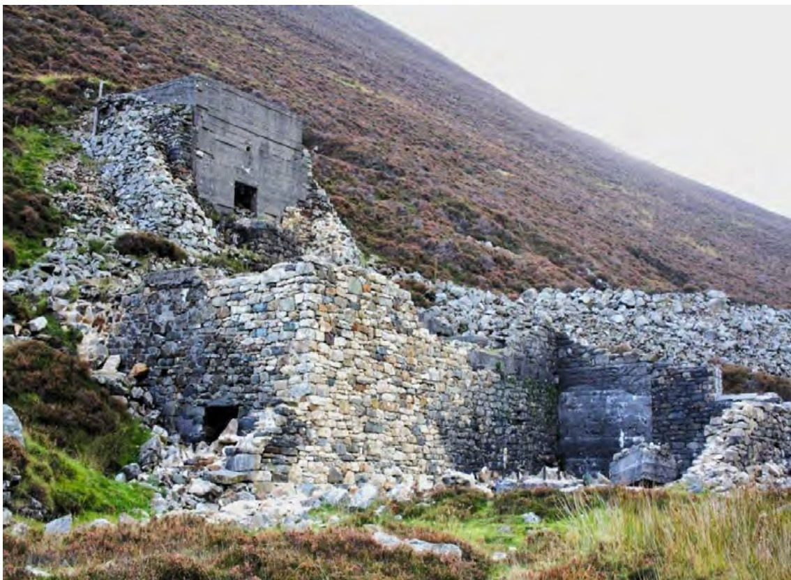
Work on the mill completed
