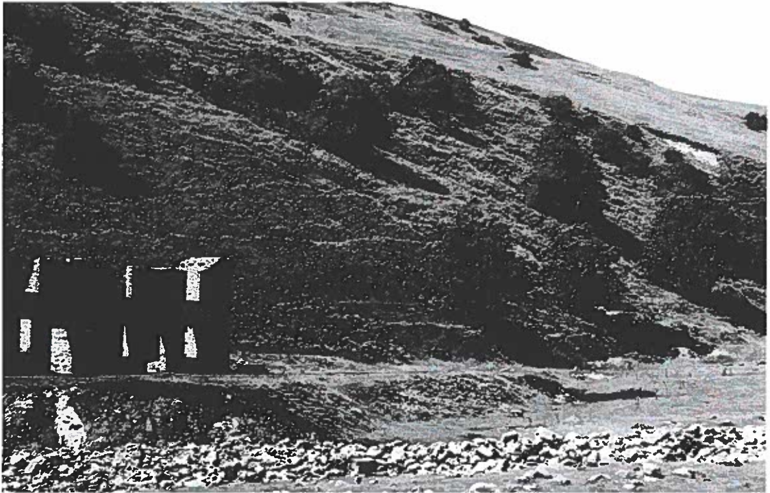
Mine building from distance. (The compressed air receiver is in the shade under the second tree right of the mine building, as is the entrance to the Sir Francis Level.)
