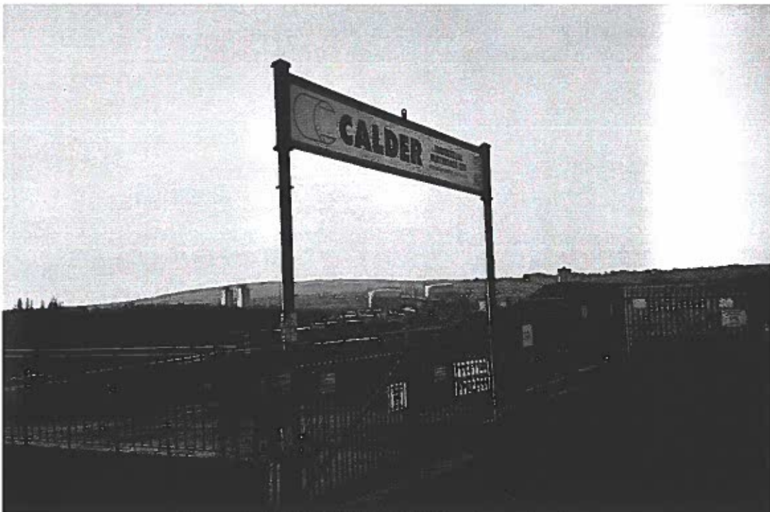
The end of an era. Calder's Elswick site cleared, January 2005
