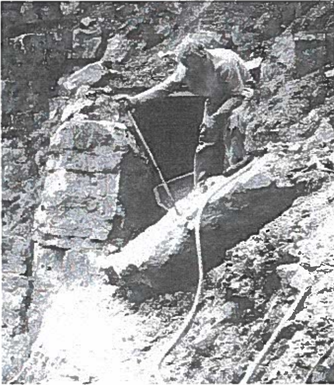
Mike Sutcliffe working at constructing a bench to access the upper fluorite-producing zone during the early 1970's.
