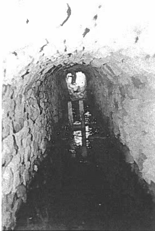
Sheaves for supporting spear rods in tunnel NY964481 Photo John Burgess
